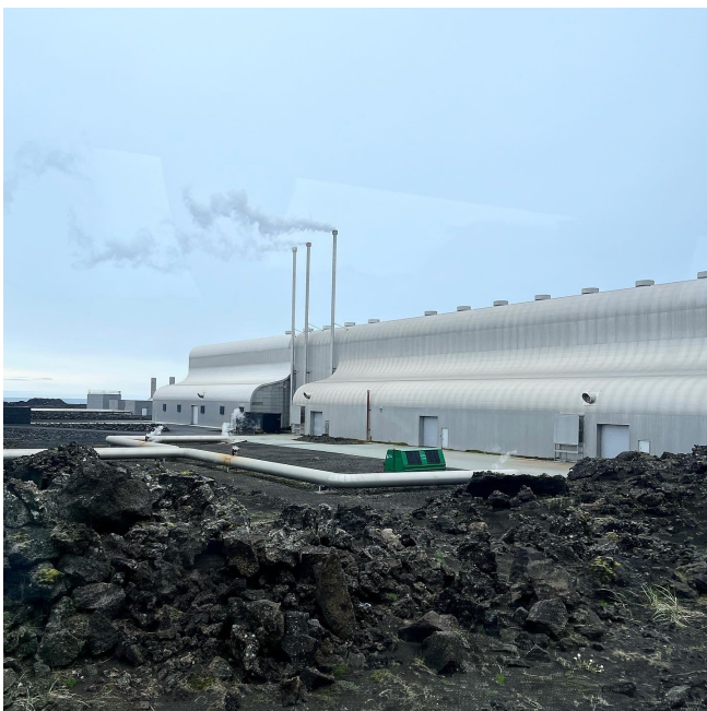
Figure 1. Reykjanes Geothermal Power Plant on the southwest peninsula.
